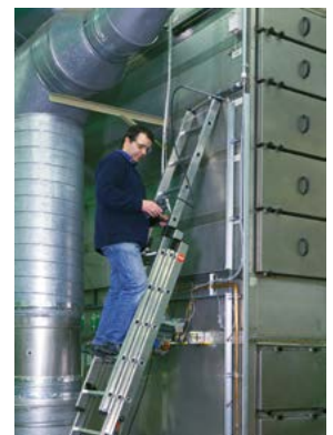
Inspecting the filter tower
