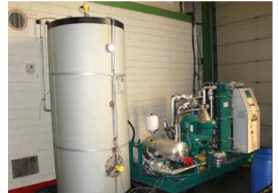
Part of the old kitchen fat heating system
