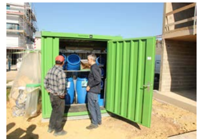
Use of the LECO box
