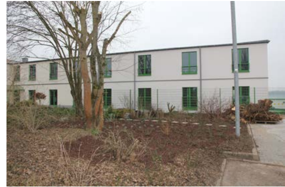
↑ The area in front of the administration building
