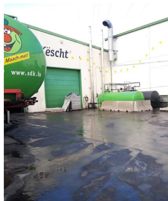
↓ Wash area with oil and grease separator
