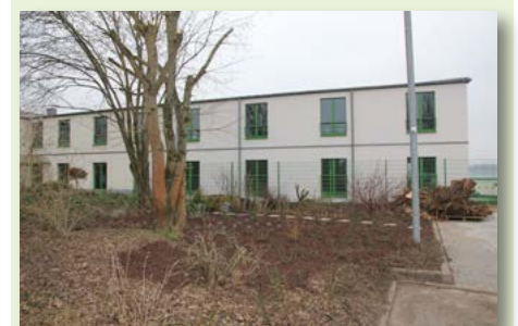
Administration building extension
