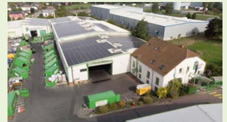
Photovoltaic (PV) system in 2022
